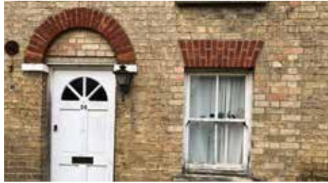
Yellow brick façades with contrasting red brick lintels.
