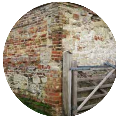
BRICK AND CLUNCH BOUNDARY WALL
