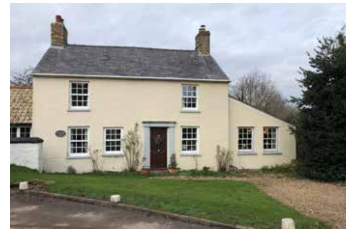
Figure 41: House with a side extension with the same treatment as the main body.
