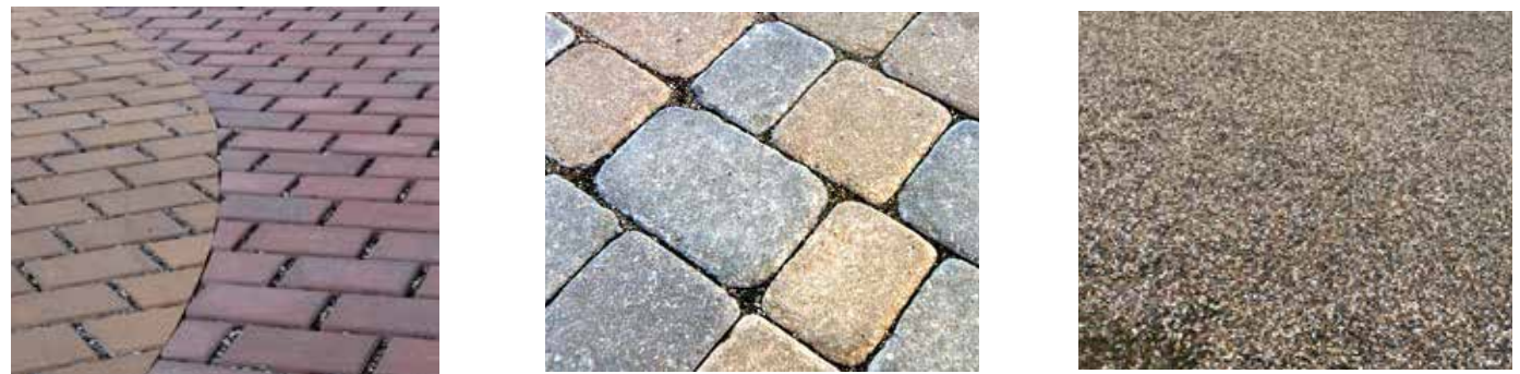
Figure 52: Examples of permeable paving treatments: clay pavers, stone/precaster concrete setts, and unbound gravel.
