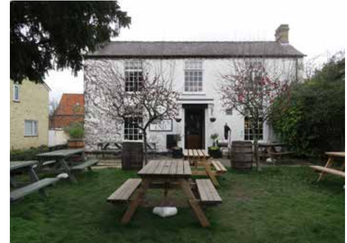
Figure 3: Dyke's End, the village's only pub on Fair Green.
