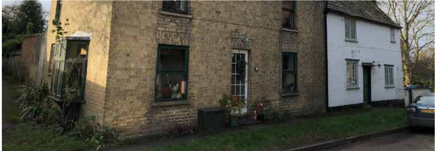
Figure 43: Windows on side elevations (left) can increase natural surveillance and sunlight inside houses.
