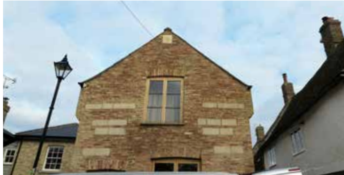
Brick and stone gable.
