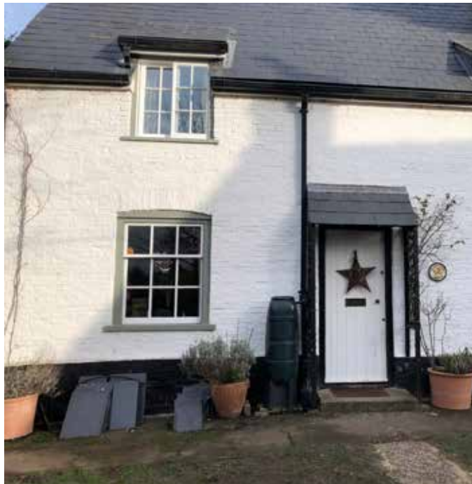
White-rendered brick house with a mix of vertical (ground floor) and horizontal (upper floor) sash windows.
