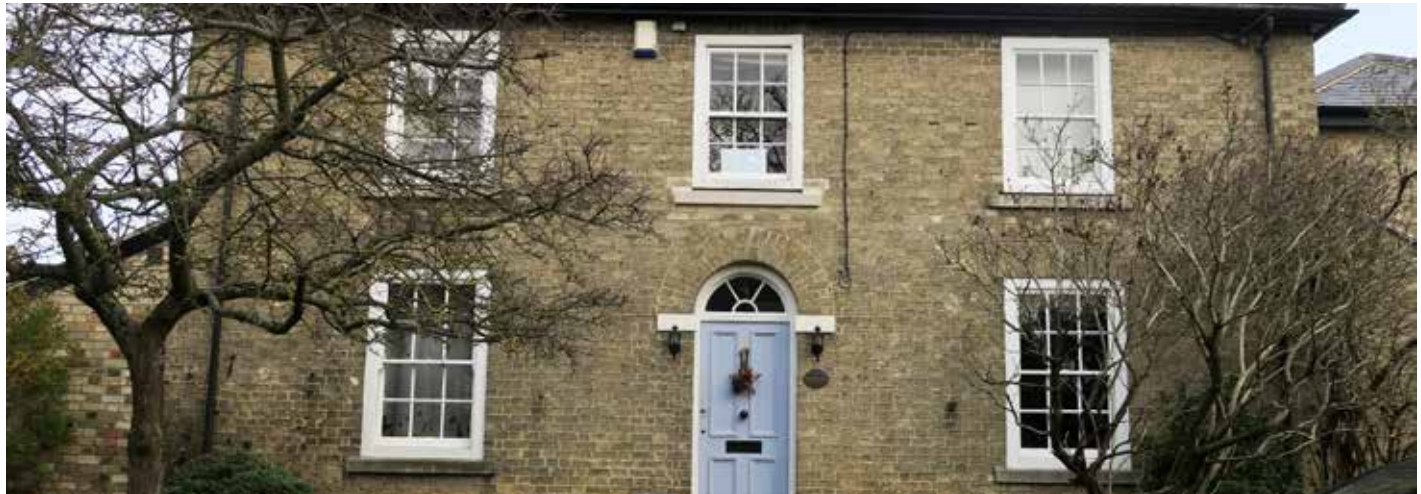
Figure 44: A façade with a simple and attractive arrangement of multi-pane sash windows and fanlight above the entrance door.
