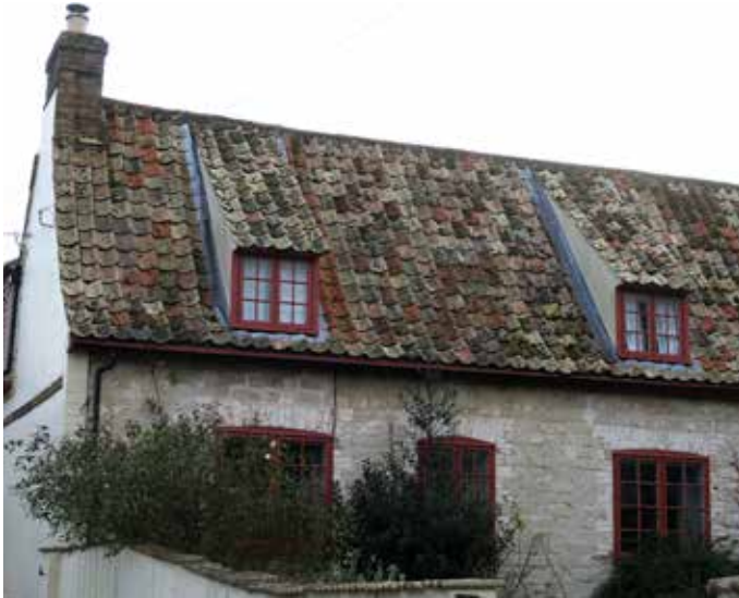
A house on Great Lane with shed dormers, clay pantile roof, and clunch walls with painted casement window details.
